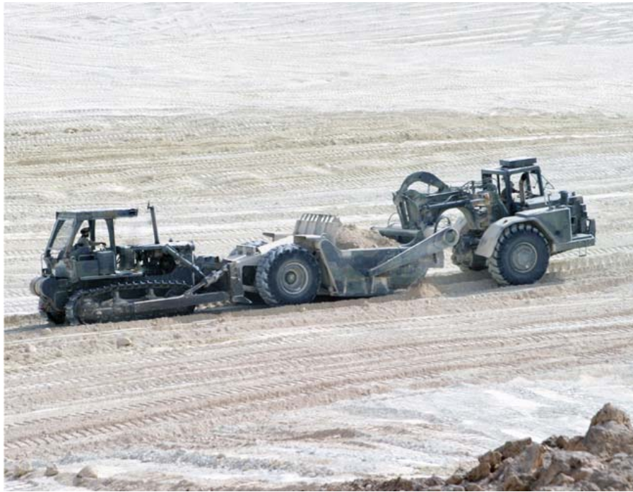
Figure 18-2 – Push cat pushing scraper.
