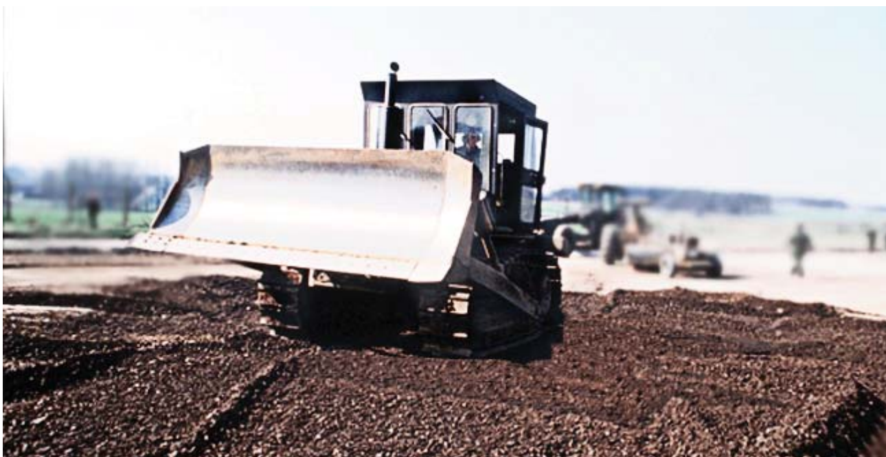
Figure 19-23 – Spreading.
