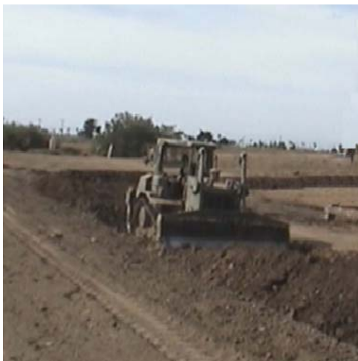
Figure 19-22 – Slot dozing.
