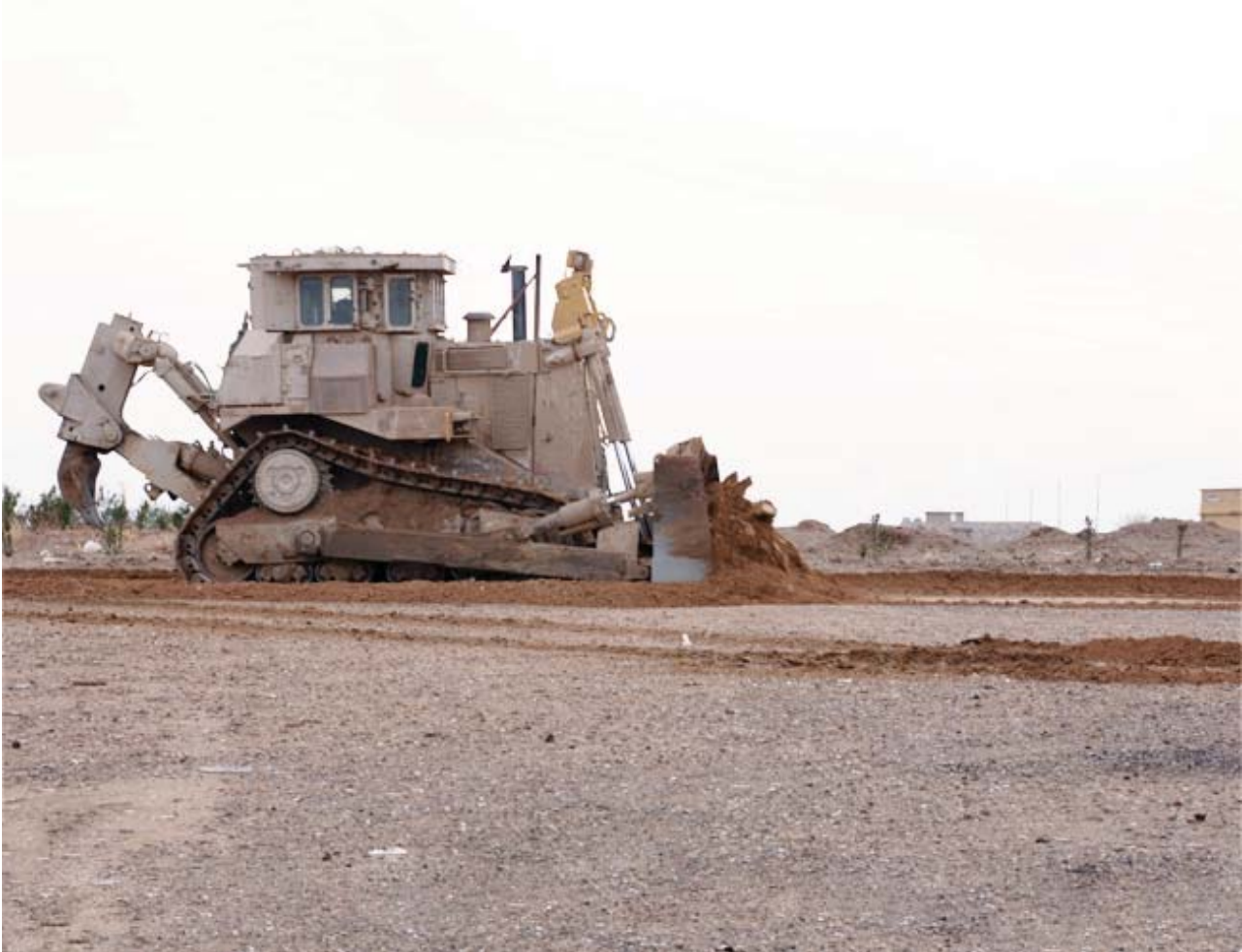
Figure 19-2 – High track dozer.
