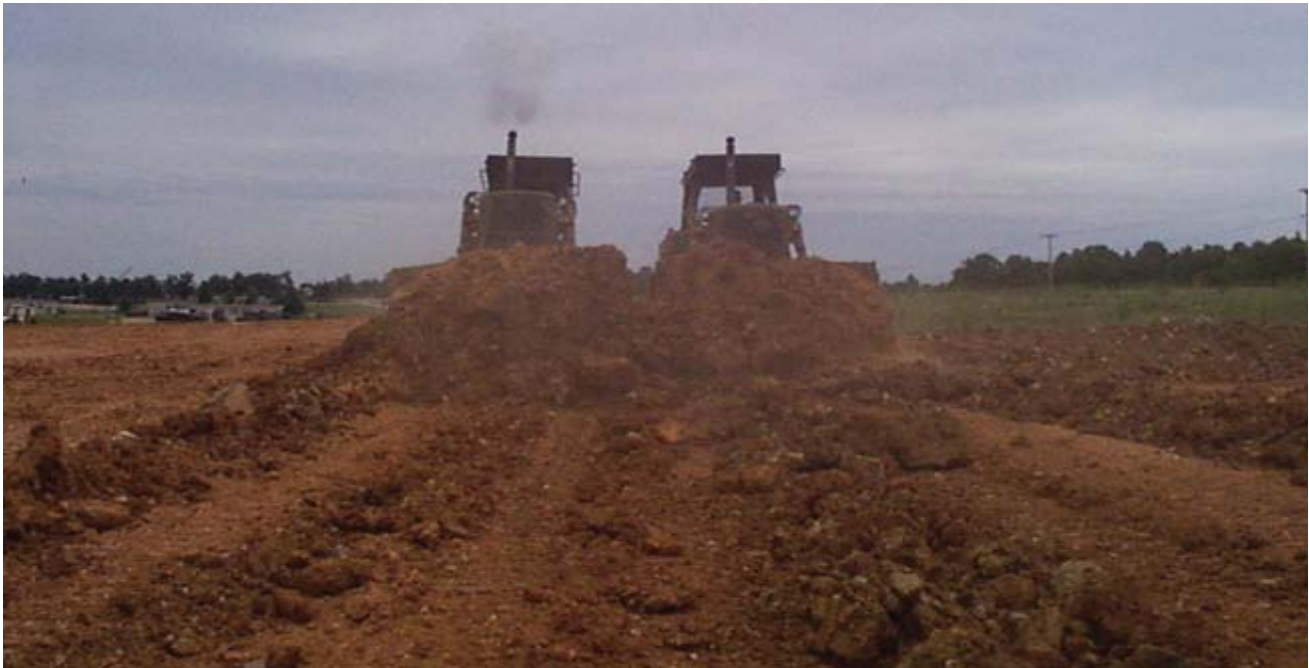
Figure 19-21 –Side-by-side dozing.
